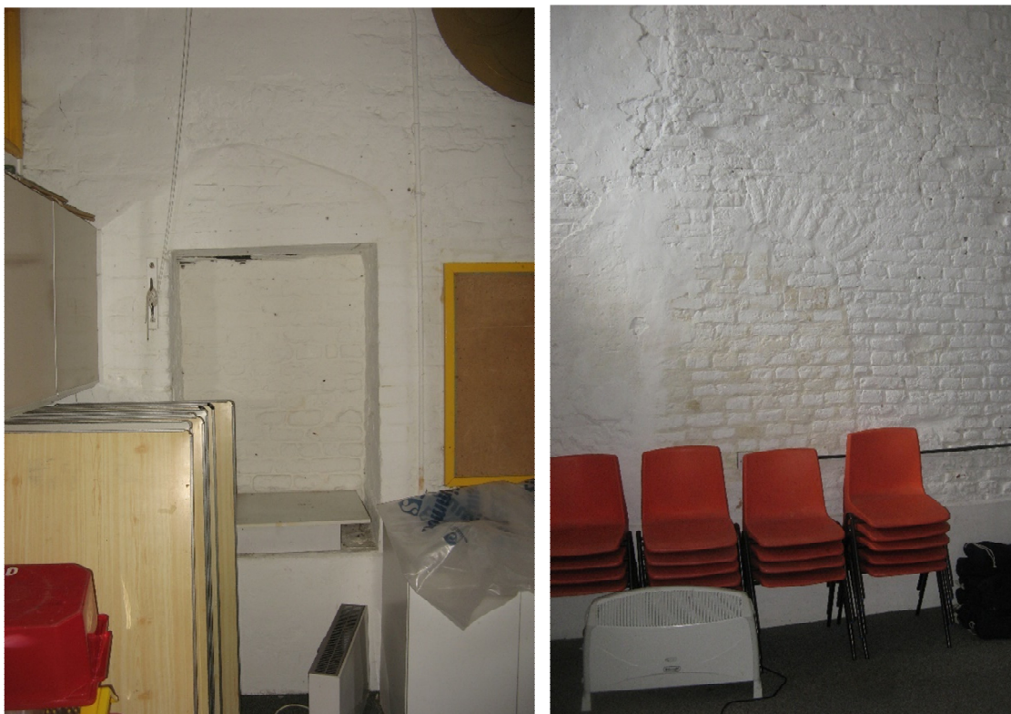
Fig 12: Gatehouse: Blocked doors from gate passage (left; for outside see fig 10) and west cloister (which appears to be secondary)
