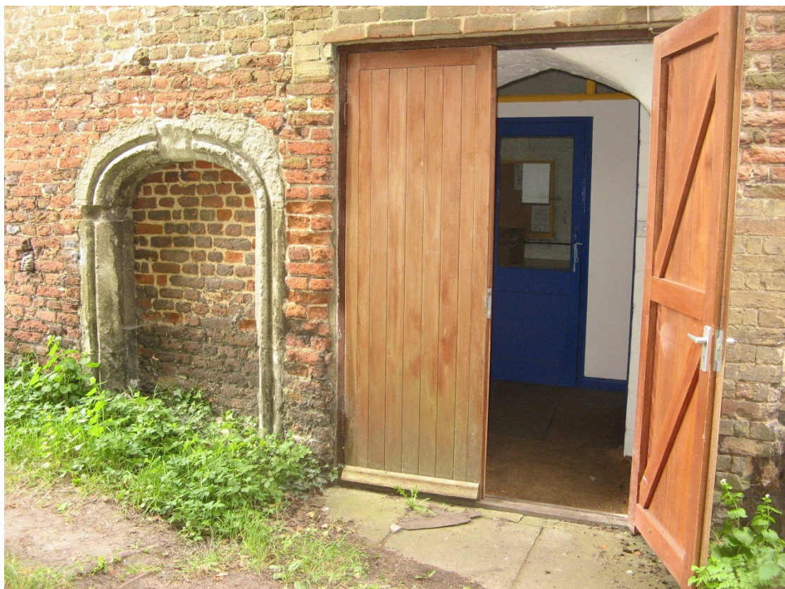
Fig 10 Gatehouse: Blocked doorway and remains of a second doorway, much altered and enlarged, alongside; floor level was originally lower
