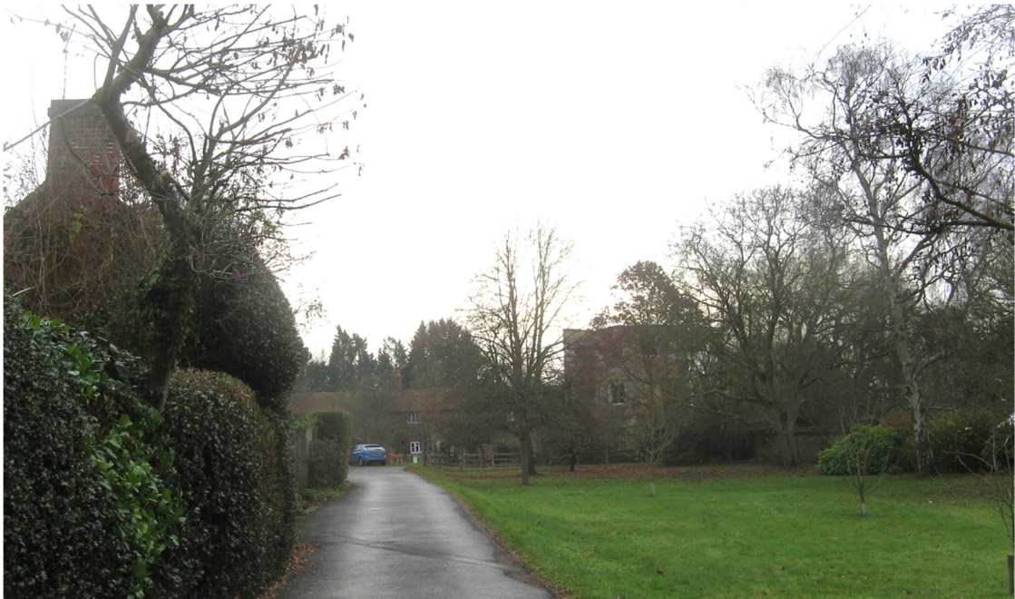
Fig 22 Castle Cottages and the north-west tower from the north; recently-planted trees in the foreground, with trunk protection still in place
